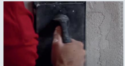
**3** Plaster can be applied approximately 30 minutes after applying SkamoEnclosure Primer.
