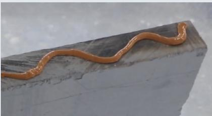
**1** Reinforce SkamoEnclosure Board joints, using SkamoEnclosure Glue.
