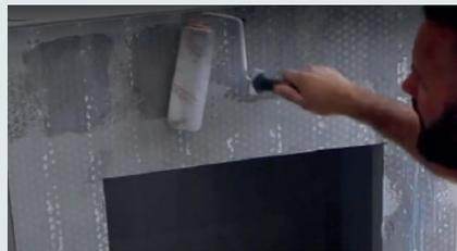
**2** Apply SkamoEnclosure Primer on the surface of the SkamoEnclosure Board where the plaster is to be applied.
