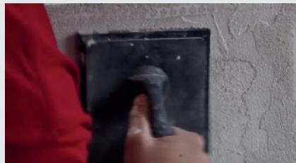
**2** Apply the plaster in an even layer thickness.
