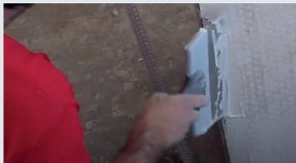
**2** Apply the plaster where SkamoEnclosure Corner is used.
