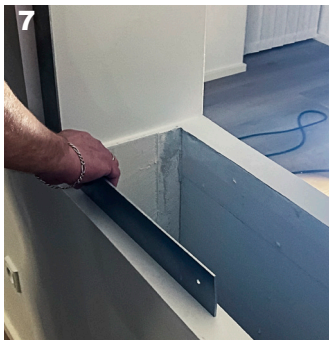
7 All cross-measures must be at an angle.
