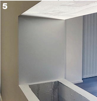
5 The fireplace wall closed at the top and sides.
